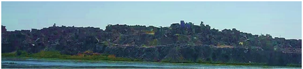
Figure 2: The front view of the Old City from the Left Bank of the river after the war. Source: Captured by the researcher
